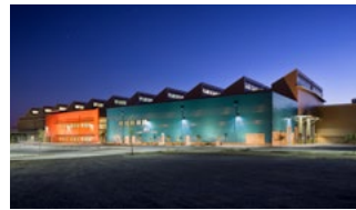
ALTAMONT COMMUTER EXPRESS EQUIPMENT STORAGE AND MAINTENANCE FACILITY
