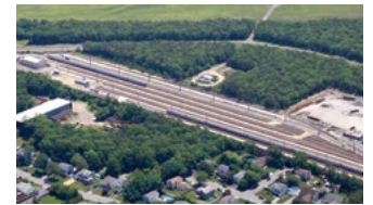
MID-SUFFOLK ELECTRIC YARD
