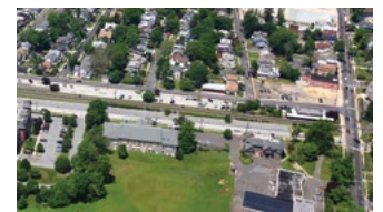
GLASSBORO-CAMDEN LINE ENVIRONMENTAL IMPACT STATEMENT Delaware River Port Authority Southern New Jersey
