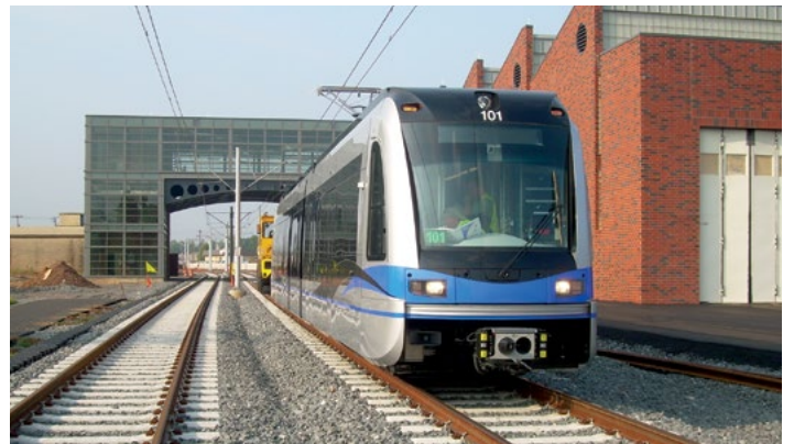
SOUTH CORRIDOR LIGHT RAIL, TRACKWORK AND SIGNALS
